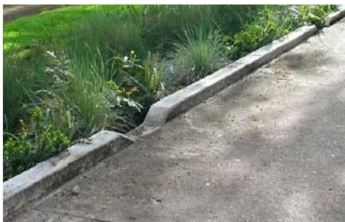
FIGURE 1 EXAMPLE OF CURB INLET
